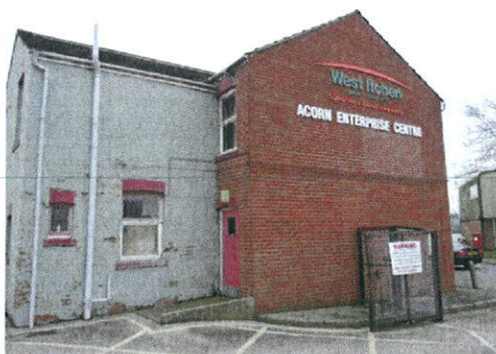
Entrance to Site and End of Terrace
