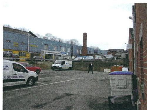
End of Site North Rear
